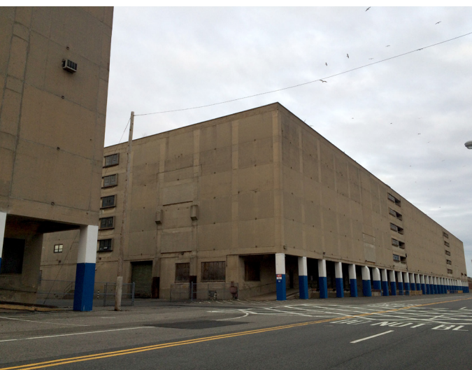
Buildings 32 and 42, now demolished, March 2016.
