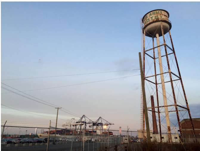
MOTBY Water Tower, March 2016.
