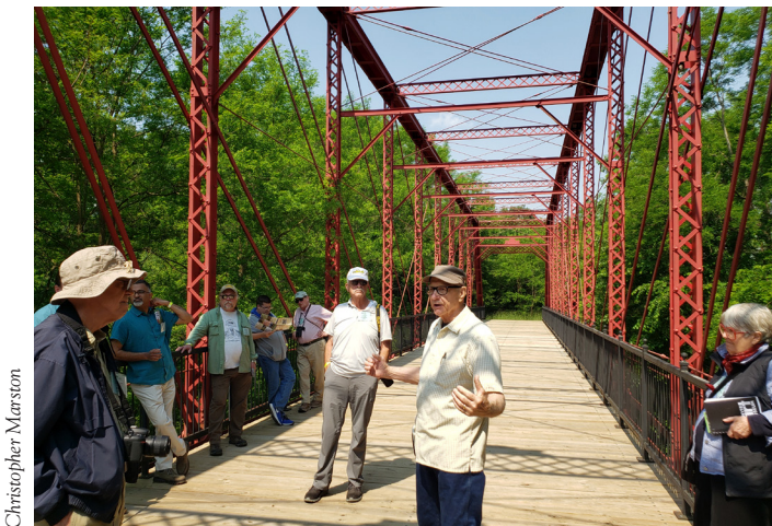
Vern Mesler describes the rehabilitation of the 1886 Charlotte Highway Bridge, a double intersection Pratt truss built by the Buckeye Bridge Co., at the Calhoun County Bridge Park.
