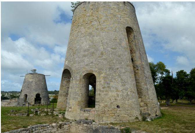
The twin windmills at estate Castle Coakley in Queens Quarter are surrounded by elaborate masonry structures to remove the crushed cane and store the cane juice.
