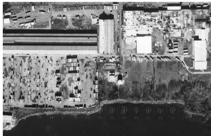
The North Yard and No. 4 Yard, ca. 1990. Remnants of No. 4 Yard shipways are awash. The north wing of the shed had already been demolished. The center section was demolished in 2022 for construction of the Delco Logistics Center.
