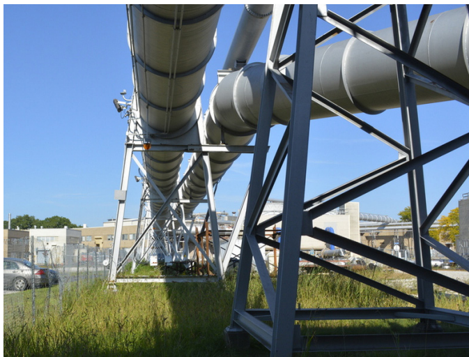
Exhaust ducts from PSL-3&4 test cells, looking from Building 64. The supply duct for the cells is the smaller-diameter line above the duct that makes the bend.
