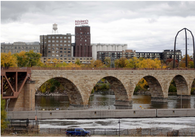
Stone Arch Bridge. Built in 1883 for James J. Hill's Great Northern Ry., the bridge crosses the Mississippi River at St. Anthony Falls. In the background left is the stone Pillsbury A Mill, built in 1881. To the right are other structures of the Pillsbury milling complex. Both the Stone Arch Bridge and the Pillsbury A Mill are National Historic Landmarks.
