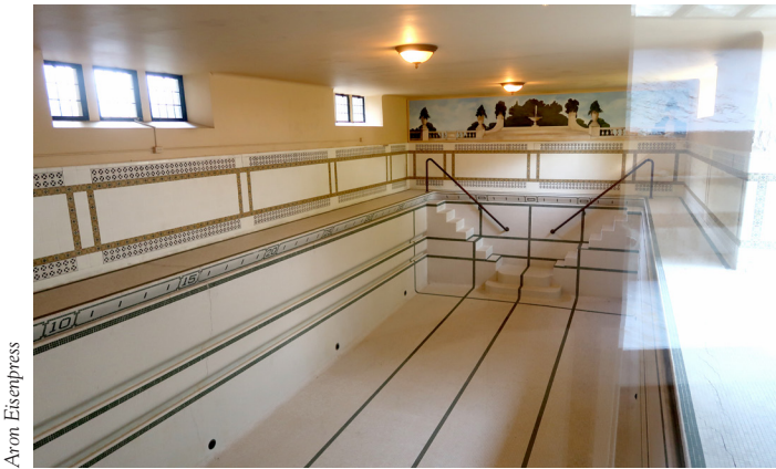
Pool (“The Plunge”) at Stan Hywet Hall. It is 46 ft. long, 16 ft. wide, 8 ft. deep, and 3’2” at the first overflow, 4’8” at the second overflow, and 7’5” at the third overflow.
