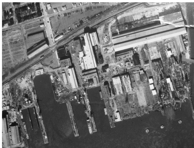
The Central Yard, now the site of Harrah's Philadelphia Casino & Racetrack, ca. 1990. A depressed floating dry dock is present in the wet basin at the bottom left. A floating crane (on the square object at the head of the smallest basin) is revealed by its long shadow. The three circular features are dolphins.
