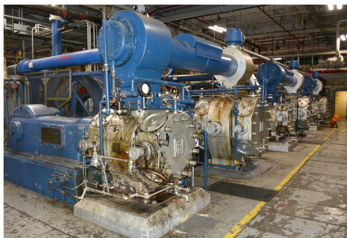
Ingersoll-Rand direct-drive duplex compound air compressors at NASA Glenn Research Center.
