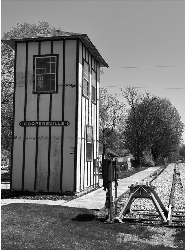
Refurbished switch tower at Coopersville. Photo courtesy Matthew Daley.
