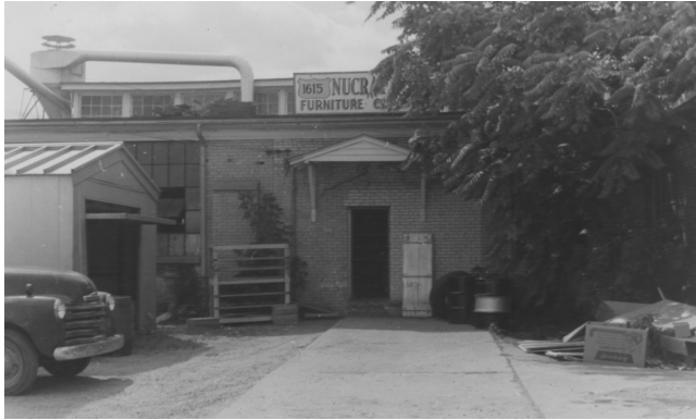
Nucraft original factory building in downtown Grand Rapids. Photo courtesy Matt Schad.
