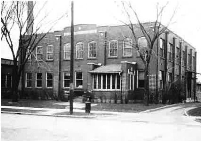
Clipper Belt Lacer office building in 1936. Photo courtesy Grand Rapids City Archives and Records Center
