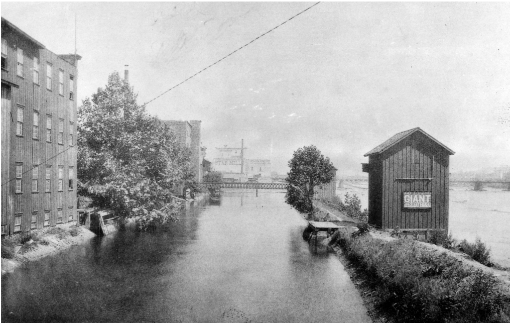
West Side Power Canal looking north from Fulton Street. Photo courtesy: Grand Rapids Public Museum.
