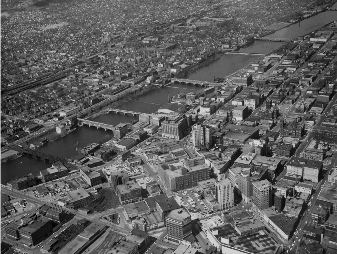
Downtown Grand Rapids looking northwest before freeway construction, circa 1955. Photo courtesy: Grand Rapids Public Museum.
