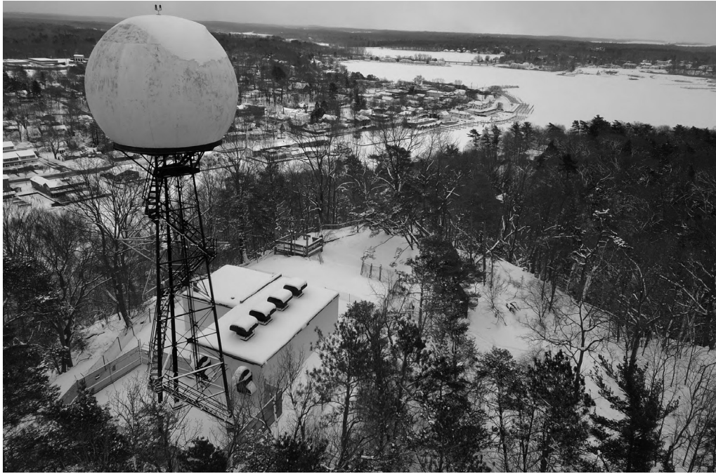
Aerial view of the Saugatuck Gap Filler Radar Annex. Photo courtesy of the Friends of the Mt. Baldhead Radar Station
