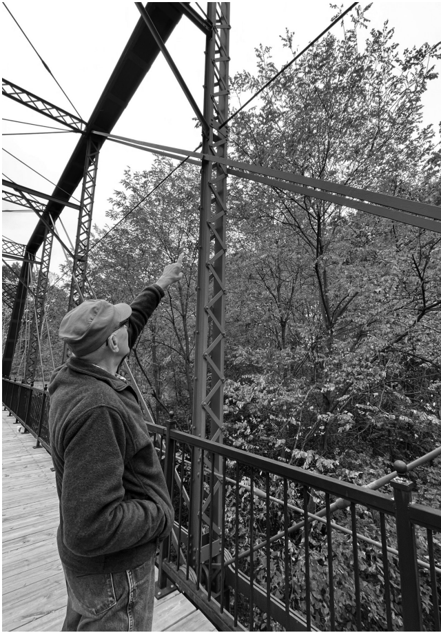
Verne Mesler leading a tour through the Calhoun County Historic Bridge Park. Photo courtesy Verne Mesler and Nan Jackson.
