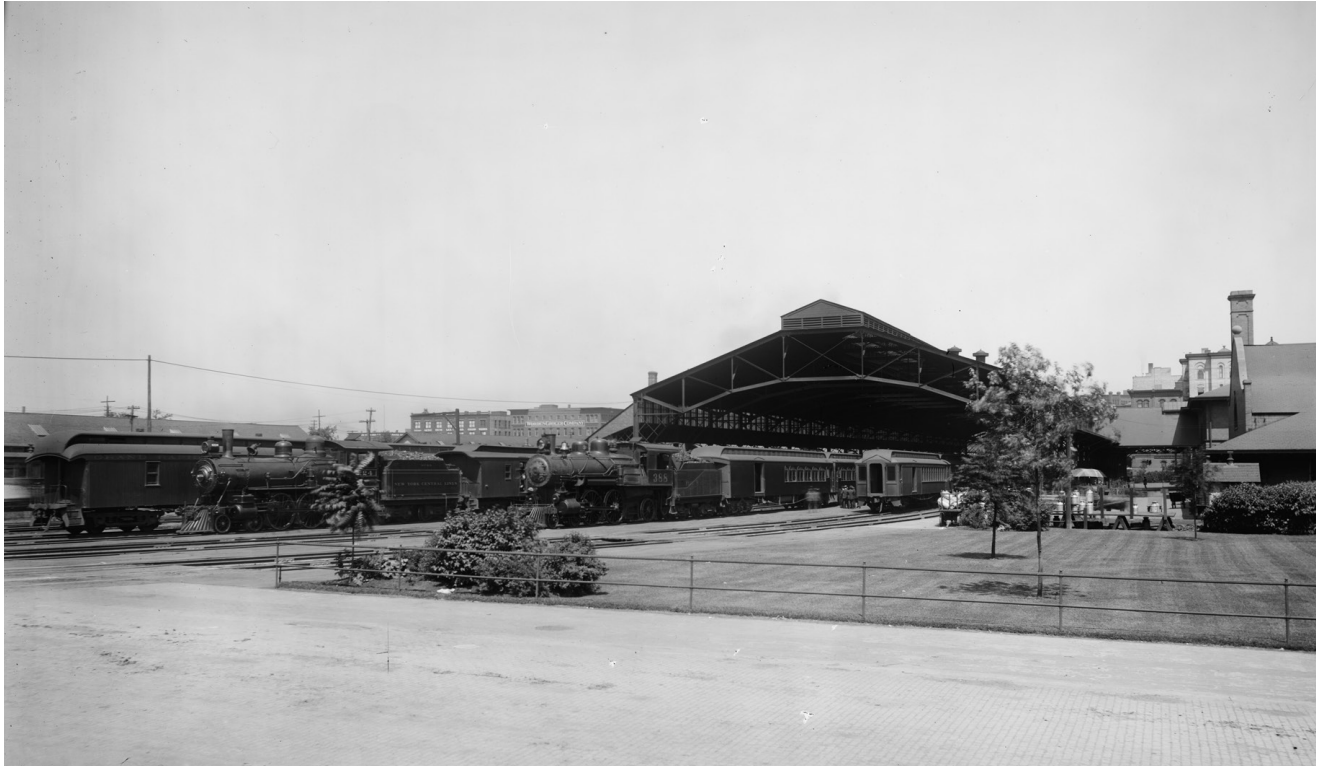
Union Depot train shed, circa 1910. Photo courtesy: Library of Congress
