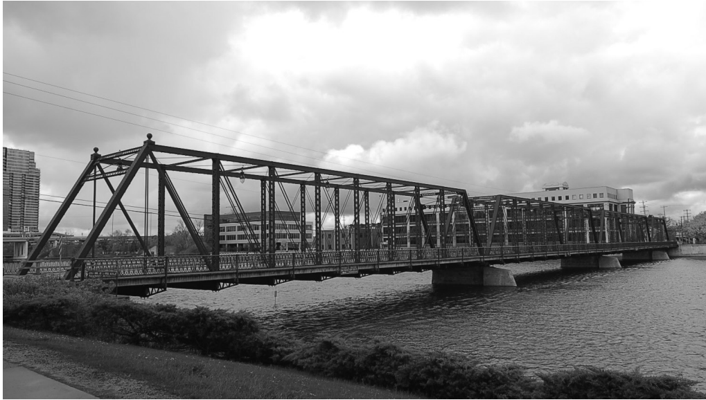
Sixth Street Bridge looking southwest in 2023. Photo courtesy: Matthew Daley.
