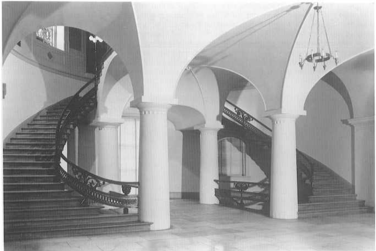
Interior view of groin vaults and cast-iron staircase of the U.S. Patent Office. HABS photograph by Jack E. Boucher, 1968.
