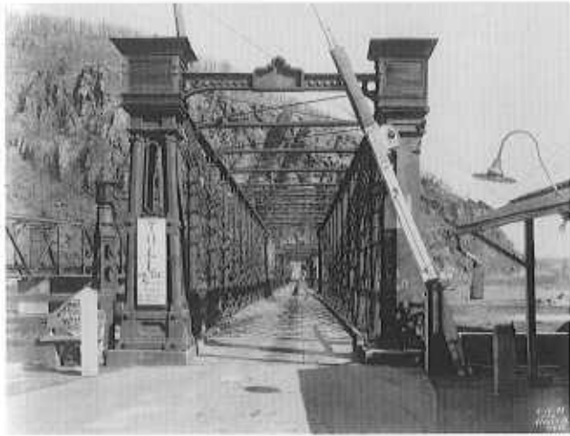
Portal of highway section of Bollman bridge, 1933, with railroad section removed. Courtesy National Museum of American History, Smithsonian Institution.
