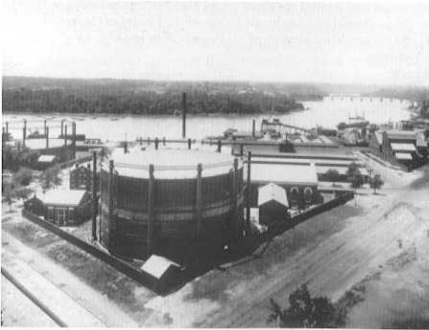
Foggy Bottom remained an industrial area well into the 20th century, as shown by the Washington Gas Light Company's West Station, on the Potomac waterfront at Virginia and New Hampshire Avenues, NW.
