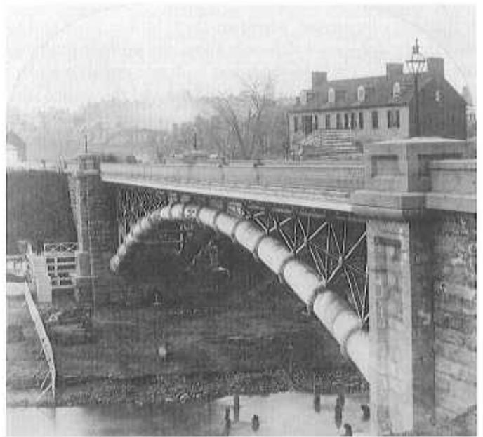
Pennsylvania Avenue Bridge, ca. 1870, looking northwest. In addition to Washington's water supply and street traffic, it carried a horse-car line. From a stereograph. Private collection.
