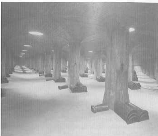
Underground slow-sand filter at McMillan Reservoir (above); Bryant Street Pumping Station interior, ca. 1905 (below). Both courtesy National Museum of American History, Smithsonian Institution.
