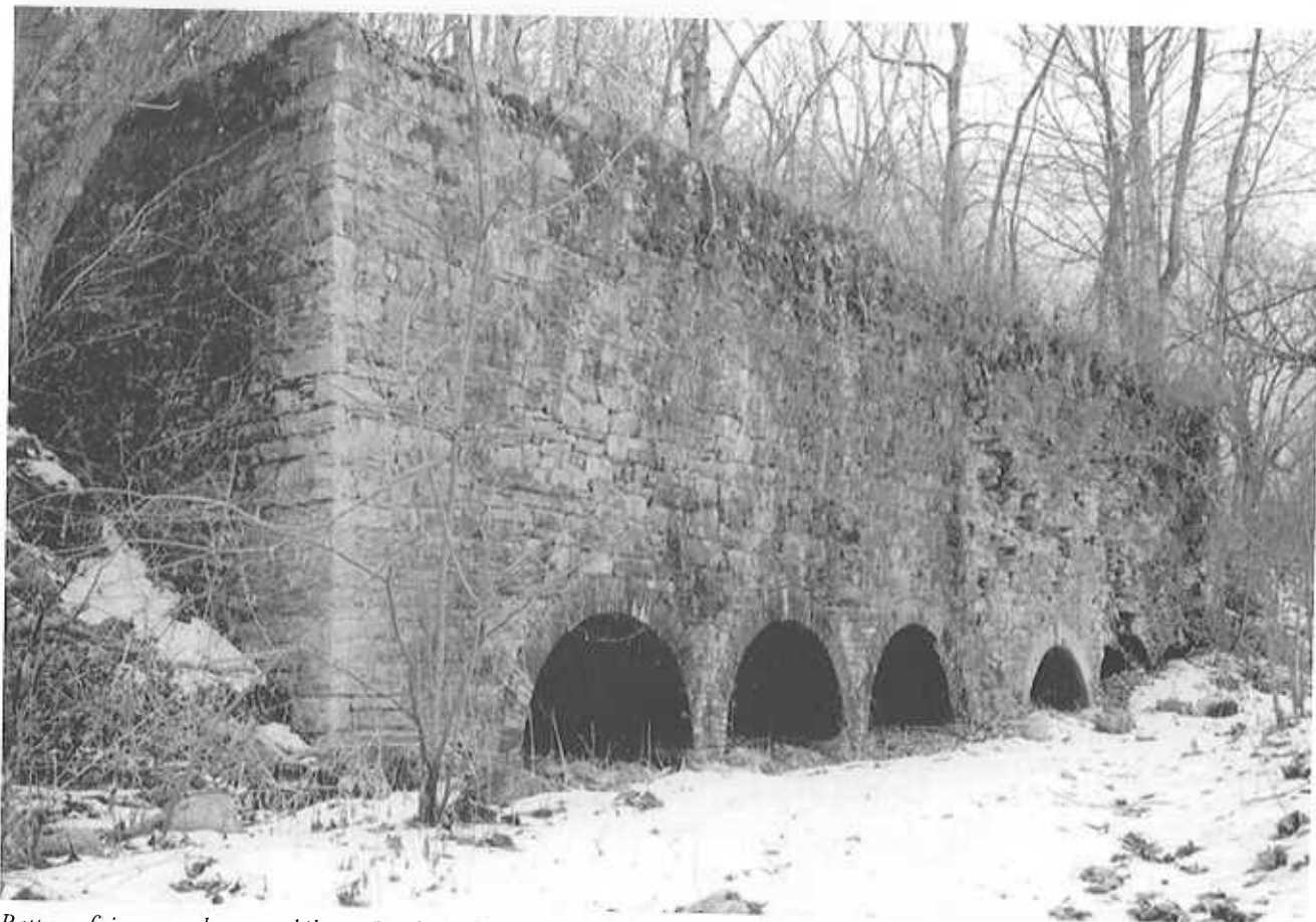
Battery of six natural-cement kilns at Boteler's Cement Mill, built 1829-30. Photograph by Christopher H. Marston, 2001.
