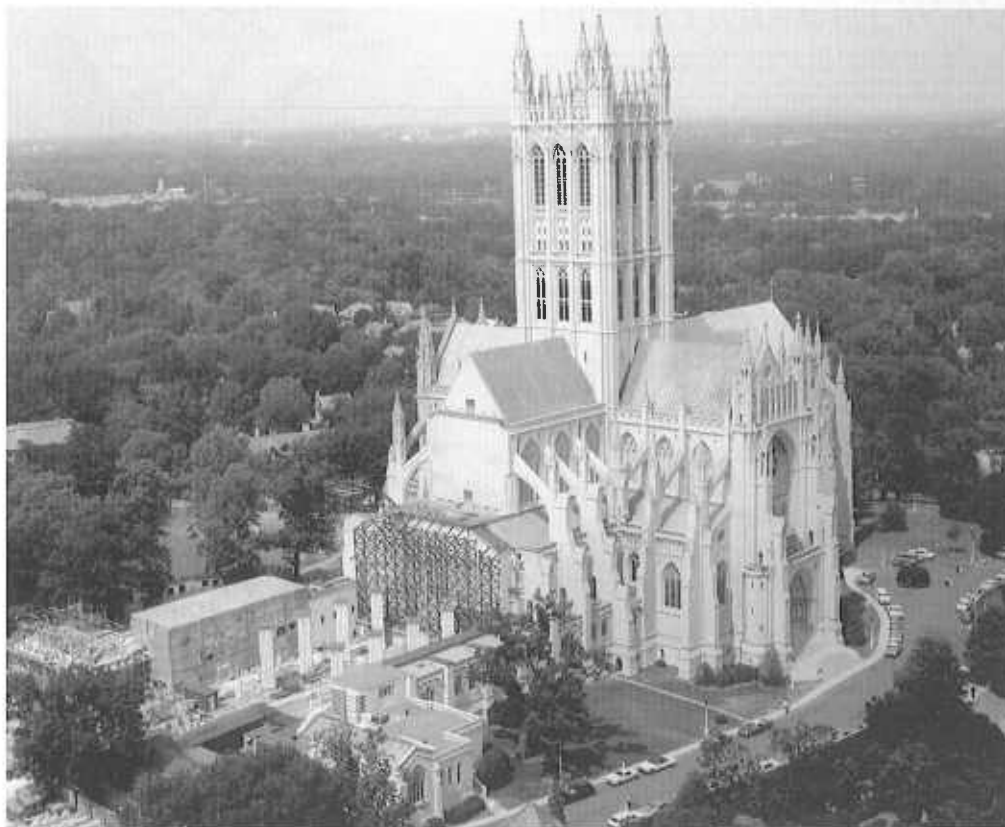
Aerial view of the cathedral under construction. Courtesy Washington National Cathedral.
