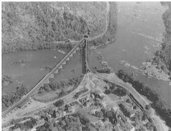
The B&O's Potomac River crossing, with its three different alignments. HAER photograph by William E. Barrett, 1970.
