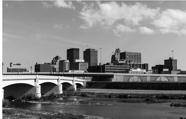
Downtown Dayton as seen from the west looking across the Great Miami River.
