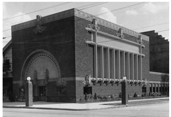
Louis Sullivan's "jewel box," The People's Federal Savings and Loan on Sidney Square.
