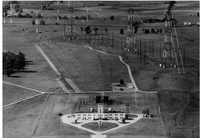
A large field of high efficiency antennas originally stood behind the Voice of America station building. Photo Courtesy VOA Museum.
