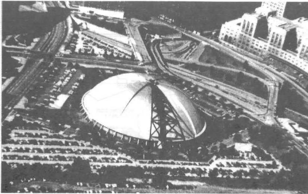
Civic Arena Auditorium Place Ammann & Whitney, engineers; Deeter & Ritchey, architects 1961
