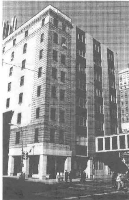
Woodwell building in its present location.
